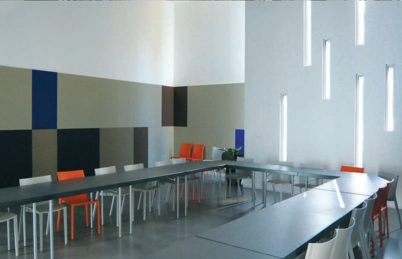
Stereo panels suspended with vertical cable fixings. Restaurant MACVAL, musée d'art contemporain du Val de Marne (Photo Hervé Abaddie) / Ripault and Duhart architecture agency, architect J. Ripault. --- Stereo panels used architecturally around the walls of a meeting room Anglet, Pyrénées Atlantiques (photo DR) / architect Philippe Pastre
